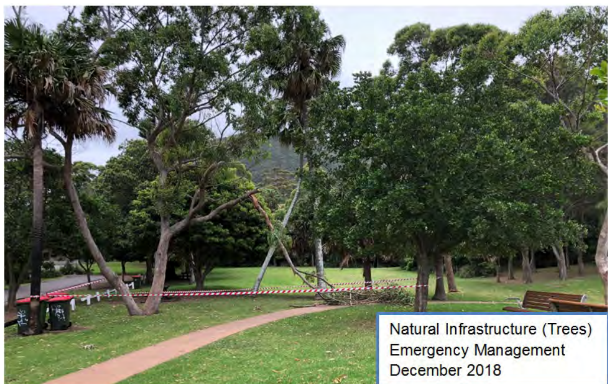
Figure 10: Example of Natural Infrastructure (Trees) Maintenance Works from Dec 2018
