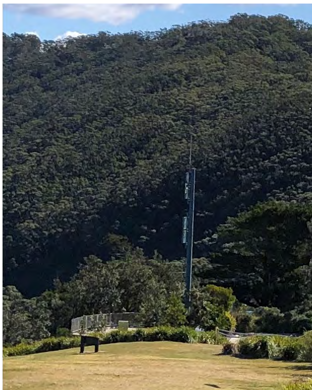
Figure 33: Telecommunications Tower at the southern end of the PoM area at Bald Hill
