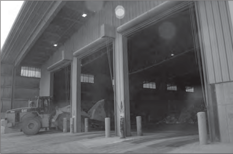
A waste transfer station where solid waste is unloaded from smaller volume collection vehicles and reloaded onto larger vehicles for shipment to landfills or other treatment or disposal facilities. Image courtesy of the author.
