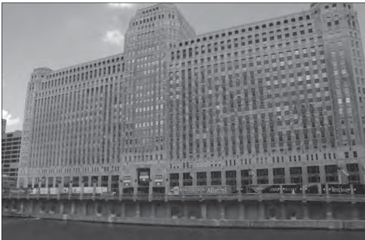
When the Merchandise Mart in Chicago, Illinois, opened in 1930, it was the largest building in the world with 4 million square feet of floor space. As the author notes, providing services (such as trash removal) to such a large structure came with its own logistics. Image courtesy of the author.
